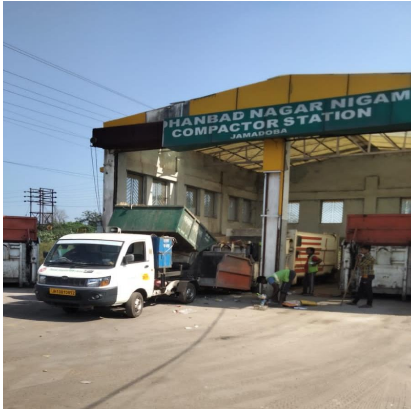
Modern Mechanized Transfer Stations at Dhanbad
